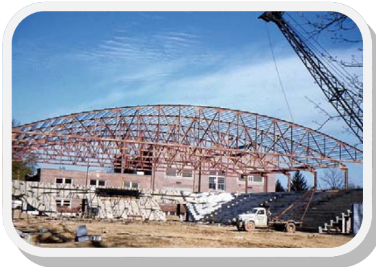
Middle School West Gym being Constructed Picture provided by Dave Hildebrand
